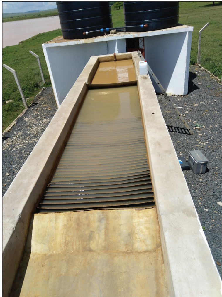
Figure 7.22: Pilot Lamella Settler Installed at Nadosoito, in Monduli District, Tanzania for Dam Water Treatment
