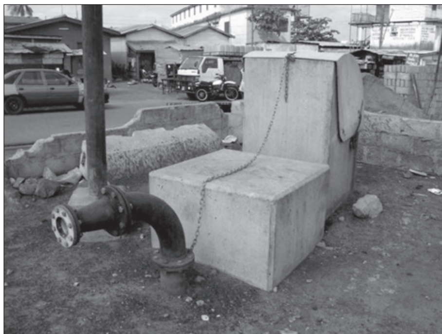
Top of an underground holding tank, showing a chain to lock the lid, a vent pipe and a wall to prevent overflowing excreta travelling onto the road
