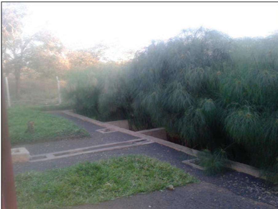
Figure 3.5: CW Treating septic Tank Effluent from Dormitory A at the NM-AIST Septic Tank-Soak-away Pit-Subsurface (French) Field Drain Combination
