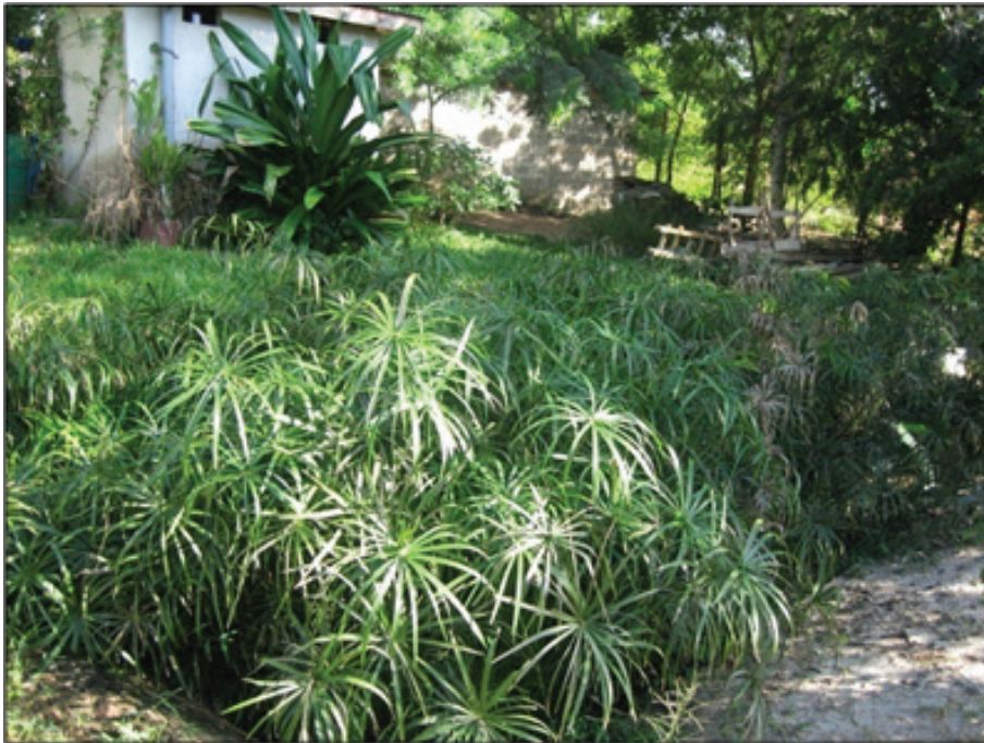
Figure 3.4: CW Treating Household Septic Tank Wastewater at Kimara Temboni in Dar es Salaam
