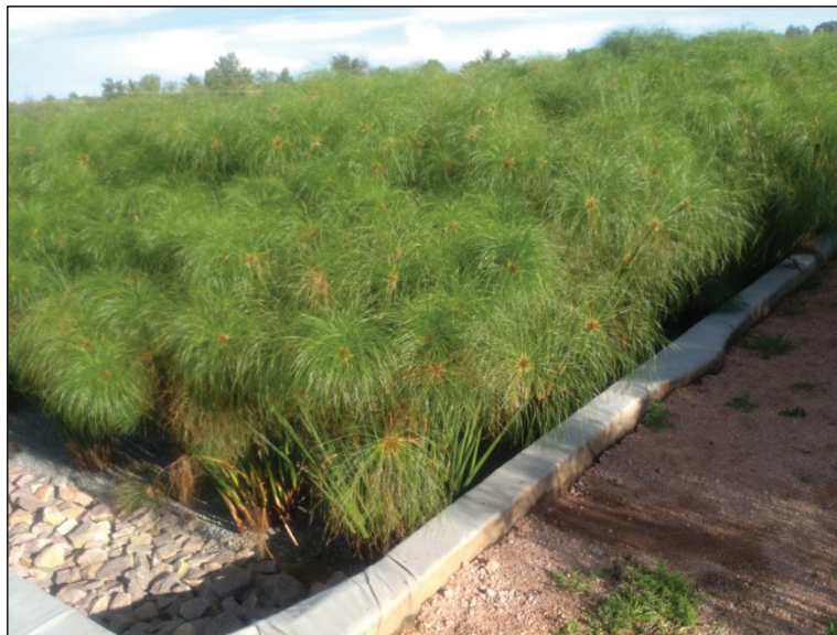
Figure 4.17: Constructed Wetland Polishing the Wastewater from Aeration Unit of Mwanza City Abattoir Wastewater Treatment System
