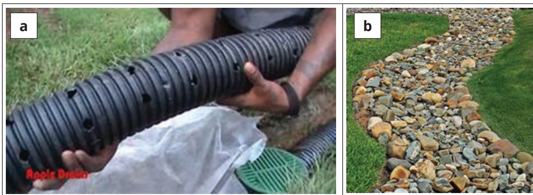
Figure 3.7: (a) Perforated Pipe for Subsurface Drain (b) Layout of Gravels
